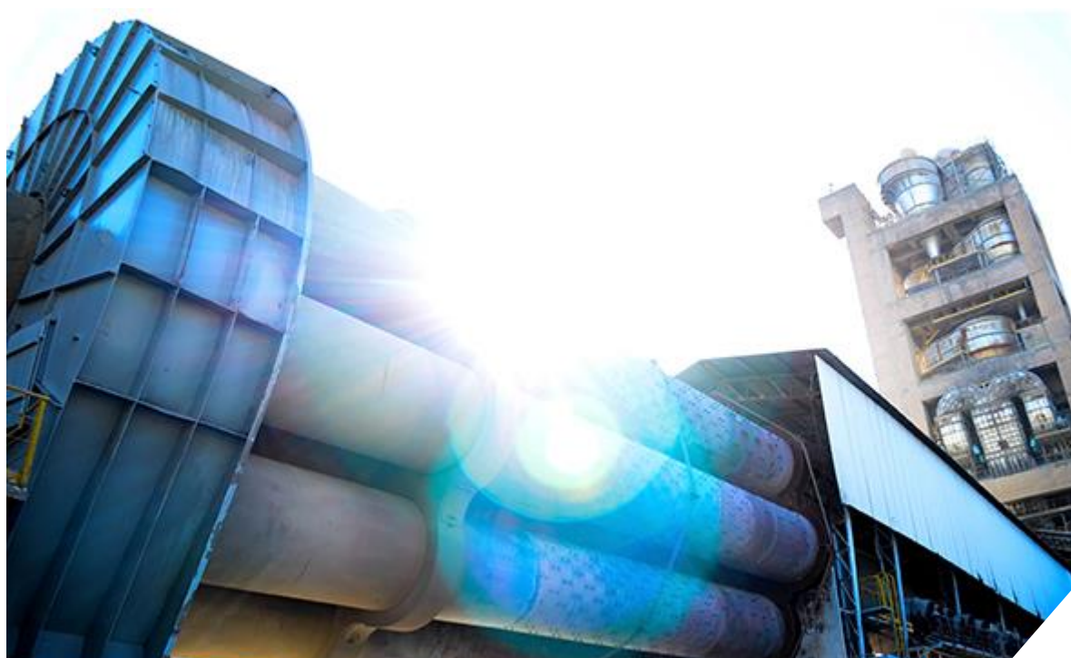
Kiln Close up – Pedro Leopoldo Plant – Brazil
